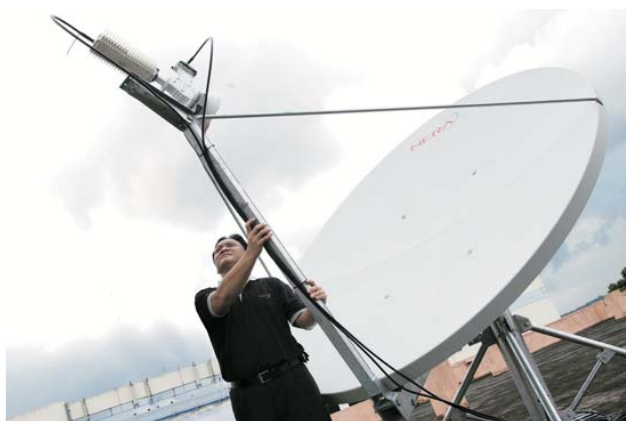
Engineer fixing the broadband satellite antenna
